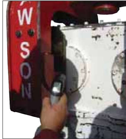
Temperature check on bearings with laser temperature gun
