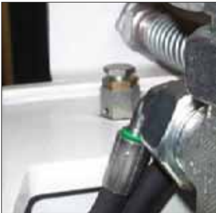
Damage to motor due to incorrect fitting of drain line
